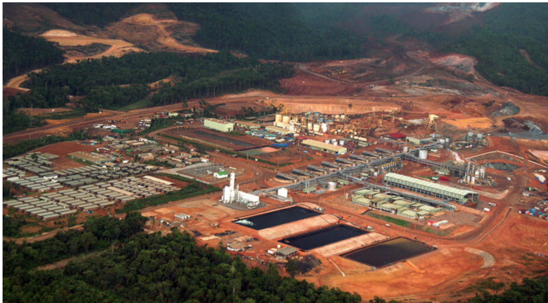
Sepon gold project in Laos. (Image courtesy of Ausenco)
